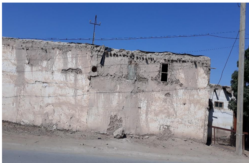
Figure 4. Exterior appearance of old houses
