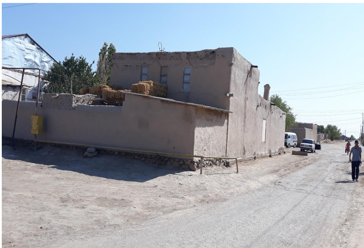
Figure 1. Exterior view of old houses
