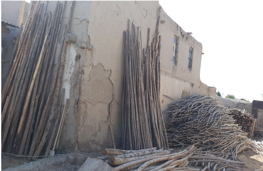
Figure 2. View of the inner courtyards of old houses
