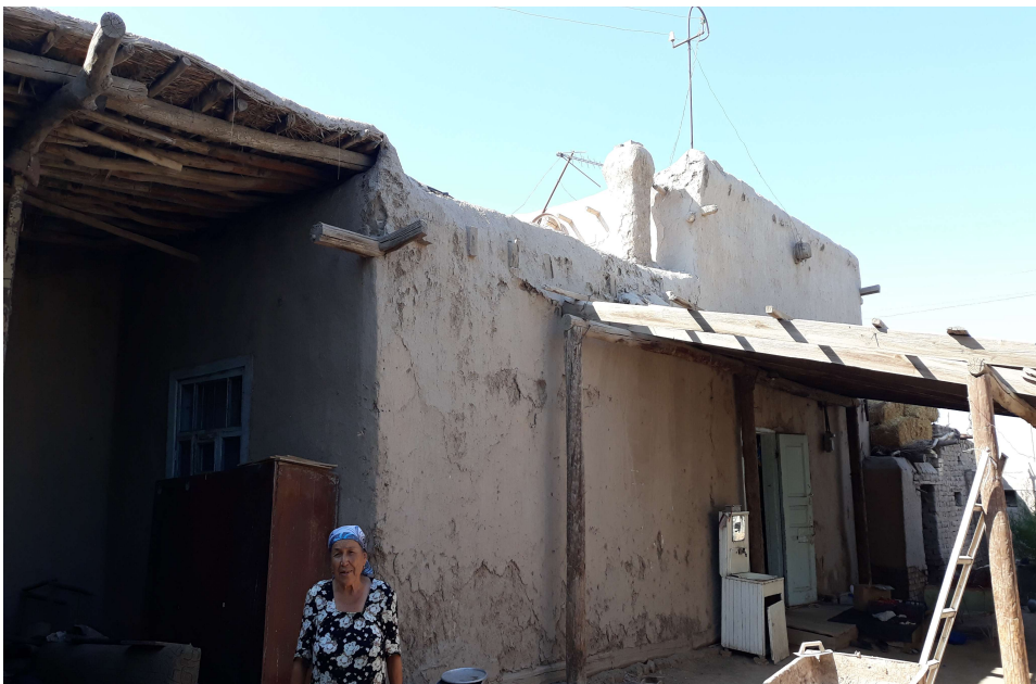
Figure 6. View of the inner courtyards of old houses
